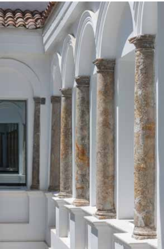
Detail of refurbished elements in the courtyard.
