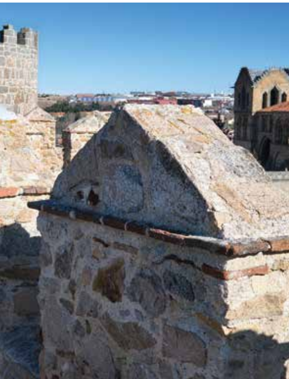
Accessible wall section.
