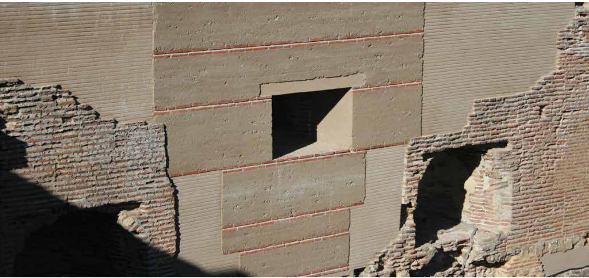
Detail of the recovered wall.
