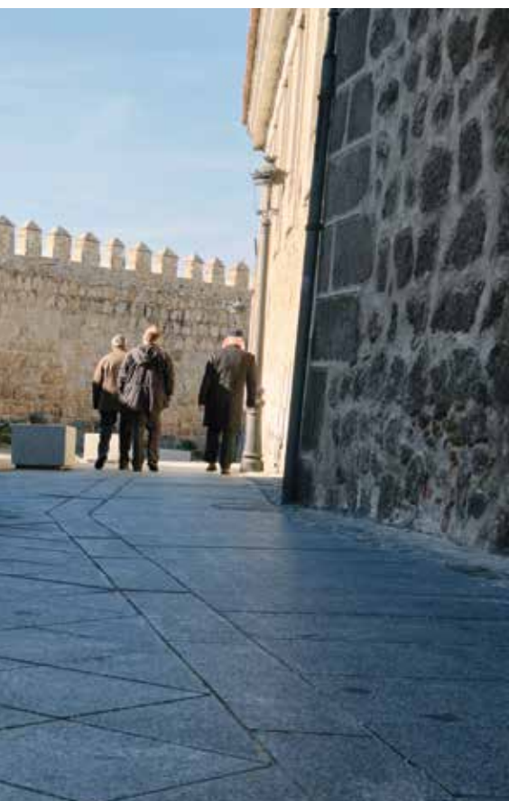
Plaza de la Santa made accessible.
