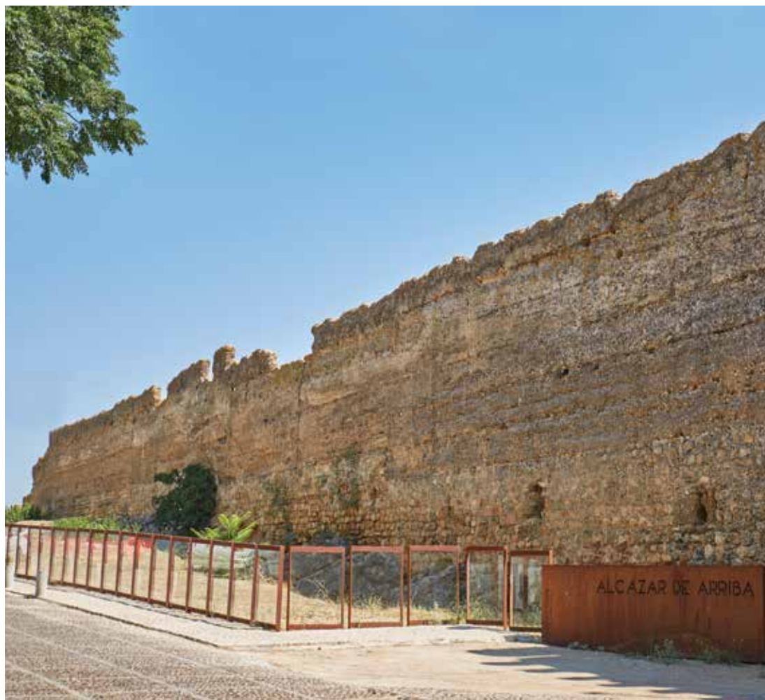
Western side of the outer wall.
