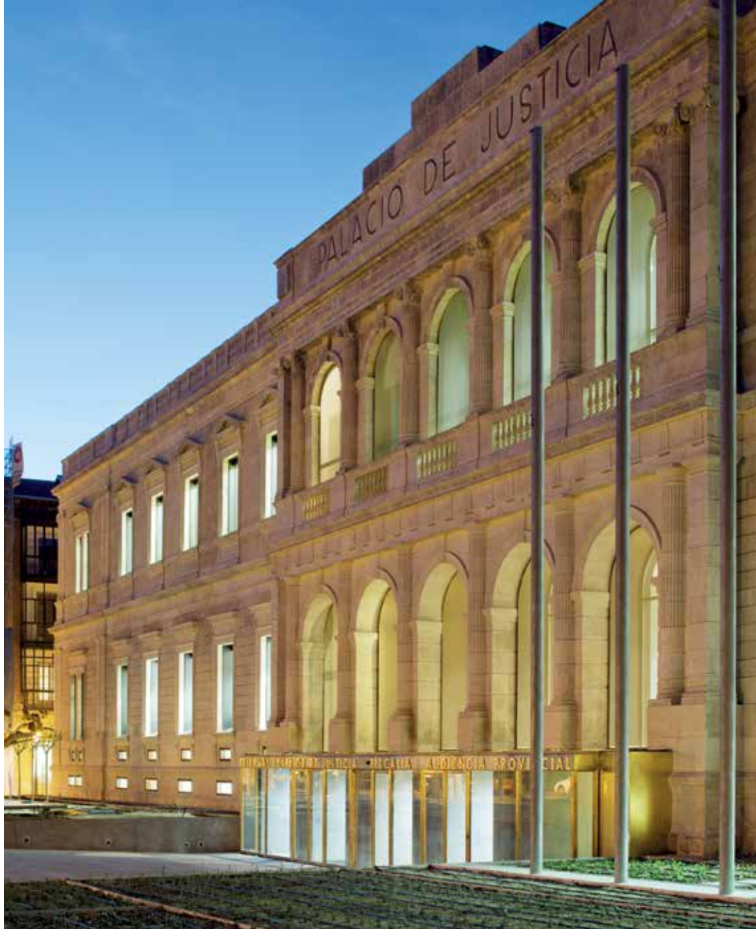
Access volume from the exterior.
