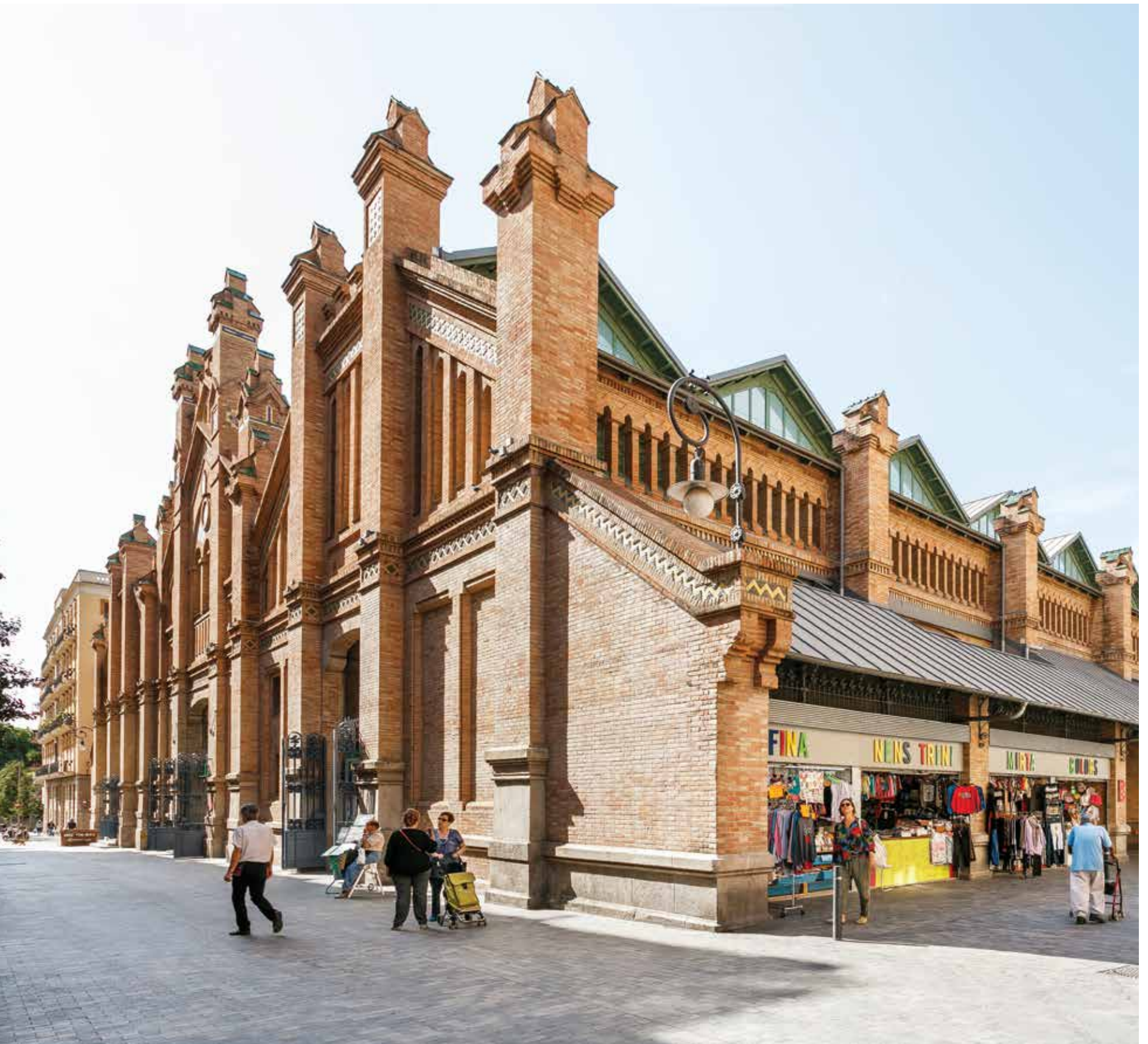
Eastern and northern façades of the market.
