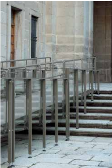
Detail of the Basilica access ramp.
