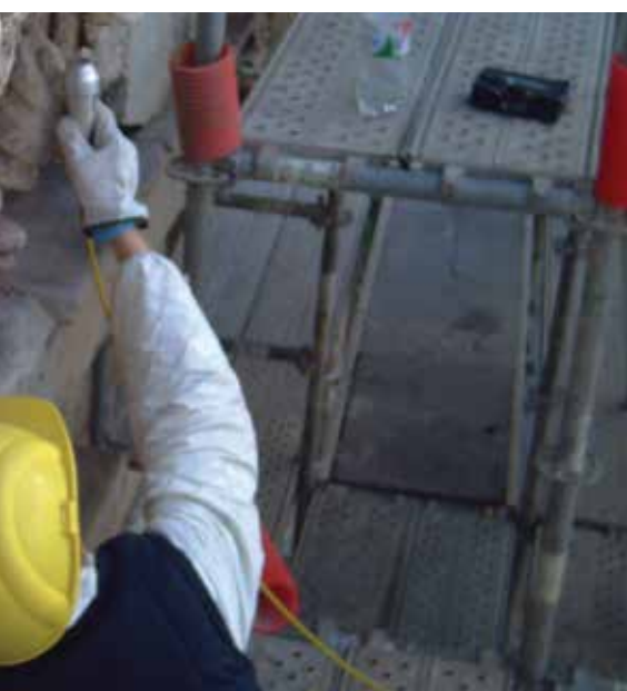
Detail of the cleaning work on the gate after restoration.
