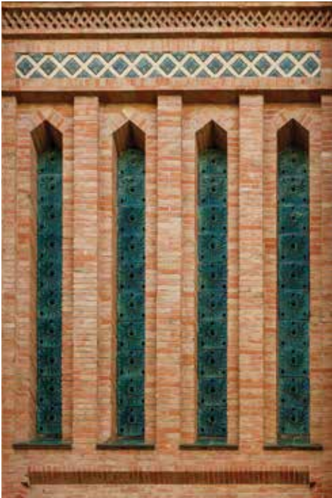
Ornamental detail of the headwalls.
