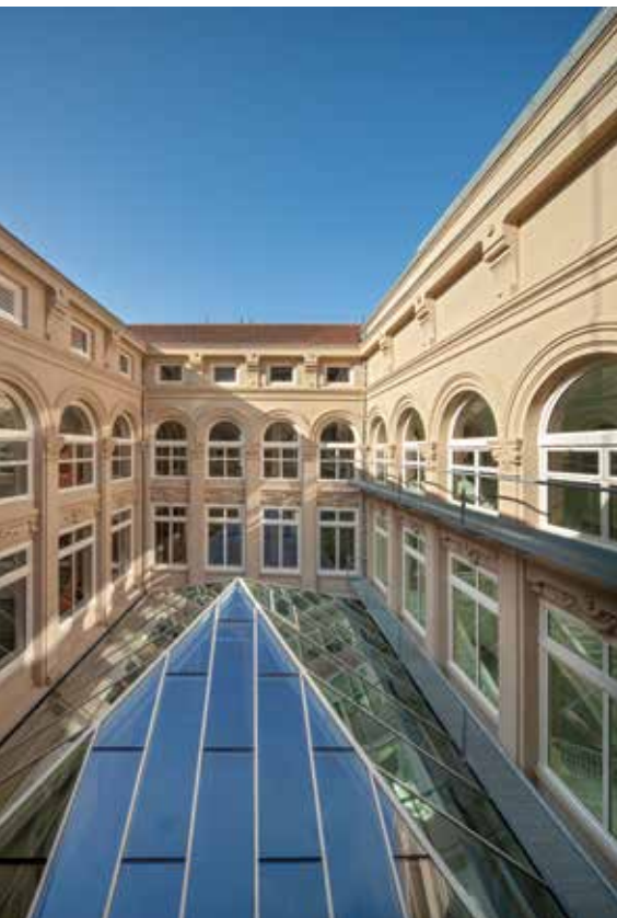
Refurbished interior courtyard.
