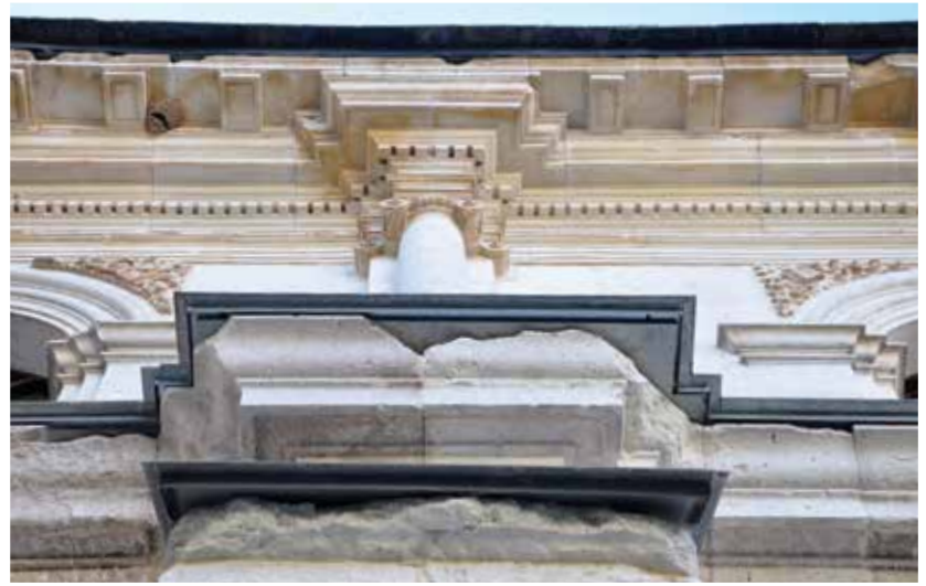
Details of the cloister façade: eaves, bays and gutters.
