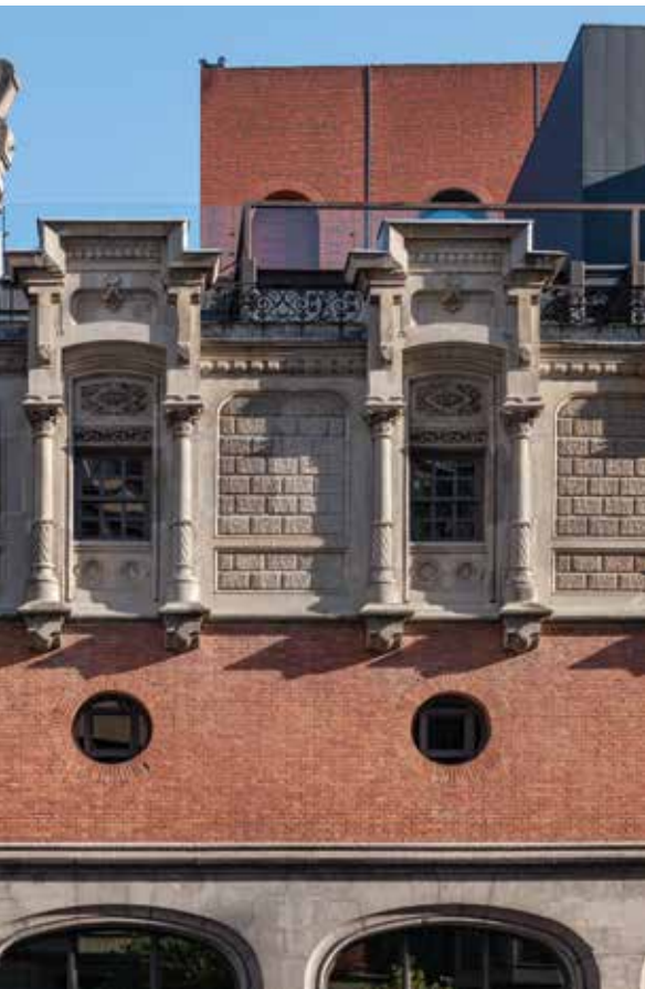
Details of the original façade.
