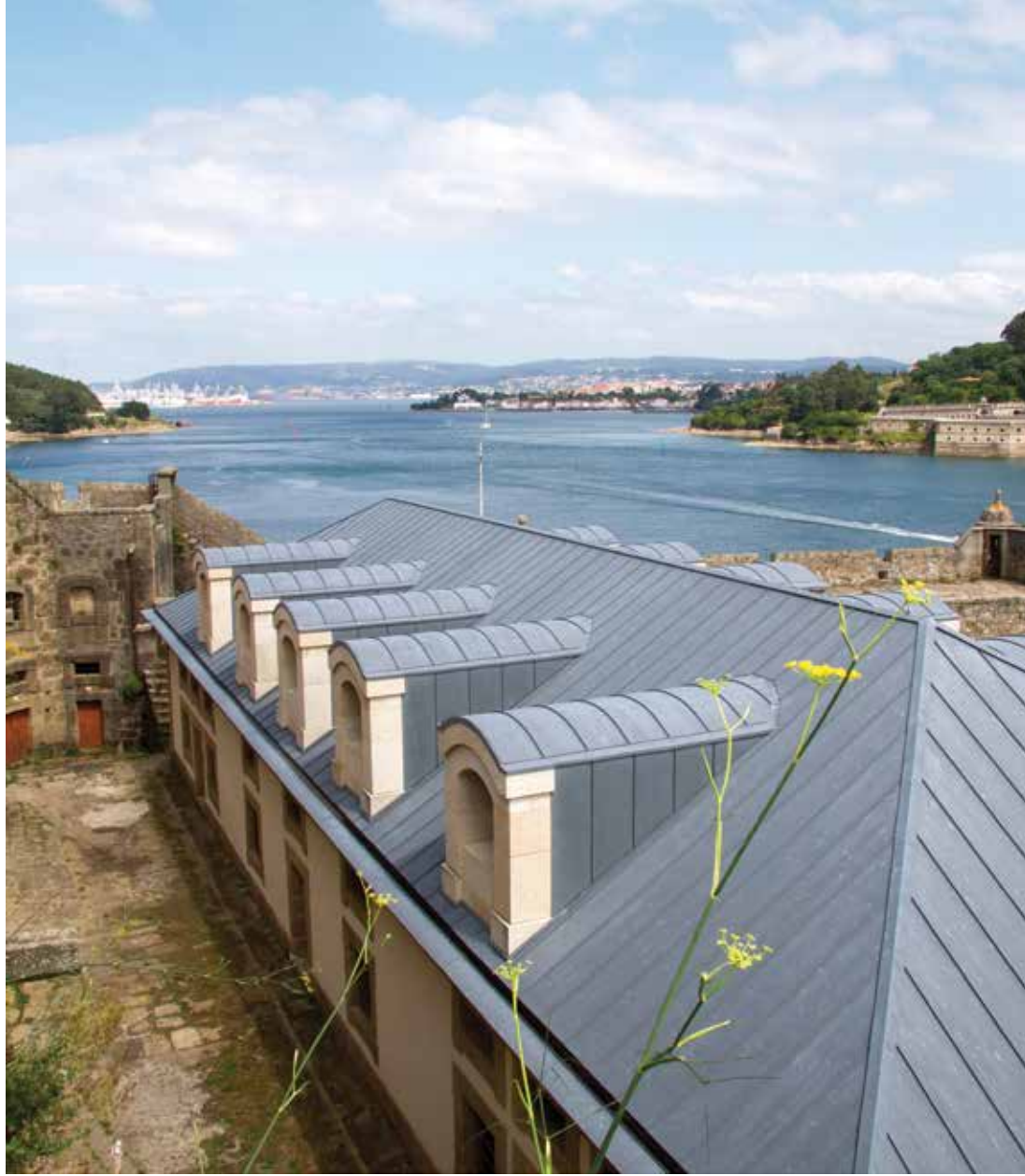
Refurbished zinc roof.
